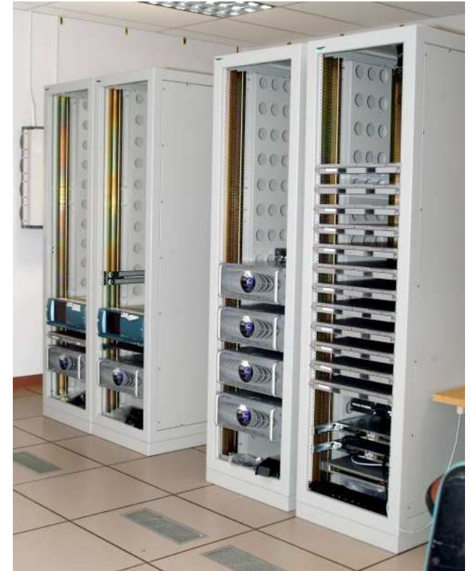
Data Distribution System being test in Building 14 (60 TB raid storage)
