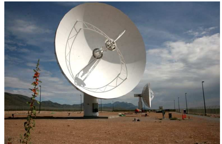
18 m antennae at STGT
