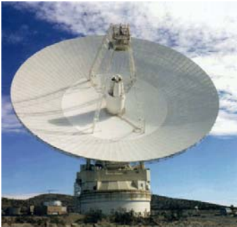
Figure 3. The 70-meter (230 feet) antenna at the Goldstone Deep Space Communications Complex in the Mojave Desert, California. This is one of many radio antennae at Goldstone, which is one of the three facilities that make up NASA's Deep Space Network. (Image courtesy: NASA/JPL)
